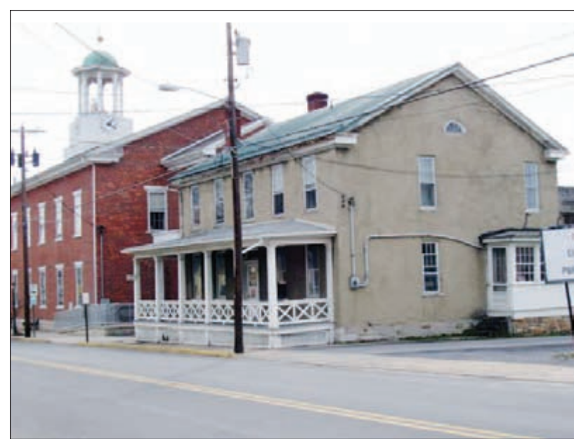
The future of the old county jail, which is listed in the National Register of Historic Places as contributing to the character of McConnellsburg, is now a concern of a statewide preservation group.
